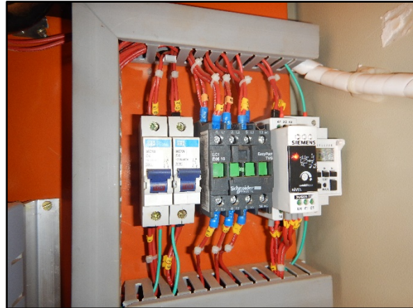
Figura 13. Chave soft start e timer digital do PT-17
